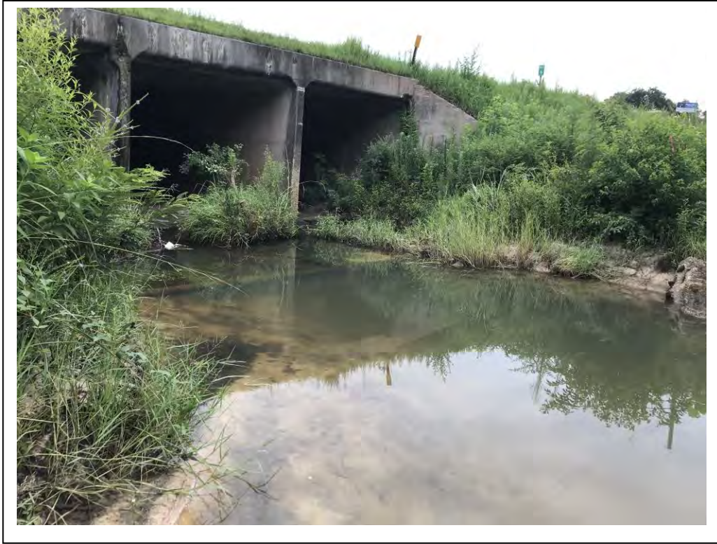
Picture #1: Norton Creek looking upstream toward Highway 43.
