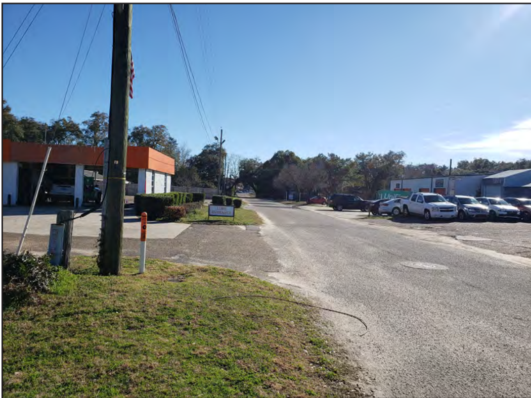
Figure 12. View of Station Street from U.S. Highway 43, facing east.
