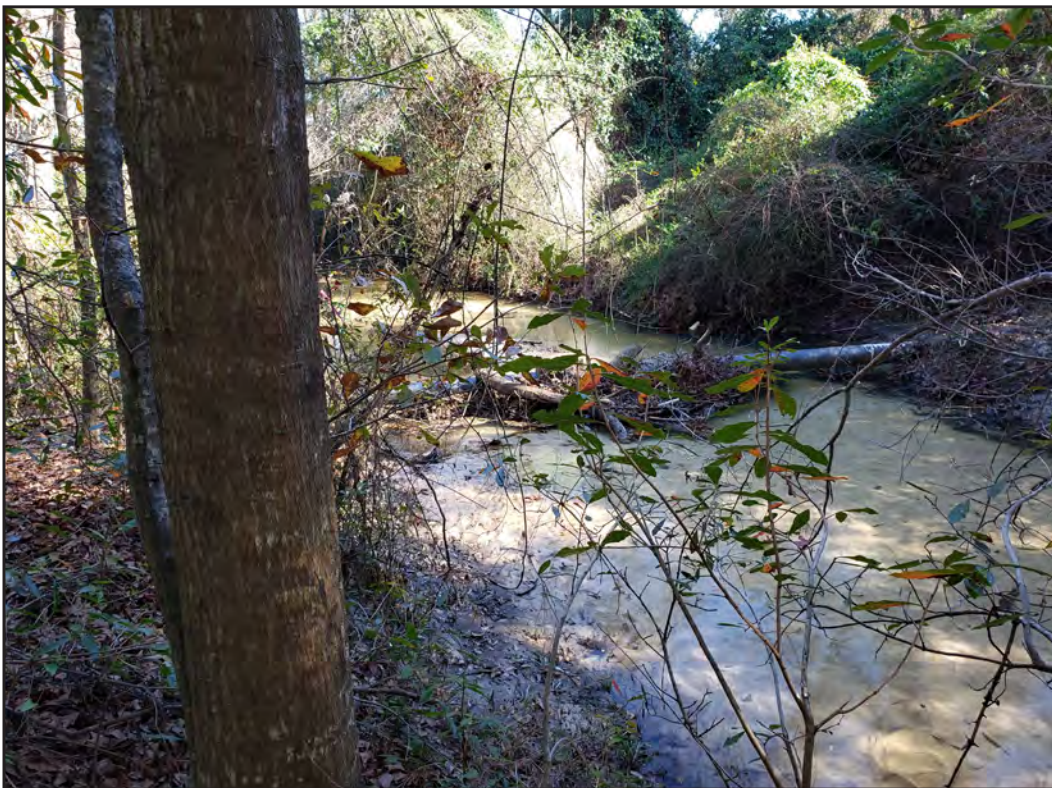
Figure 8. View of pipe crossing Norton Creek, facing east-southeast.
